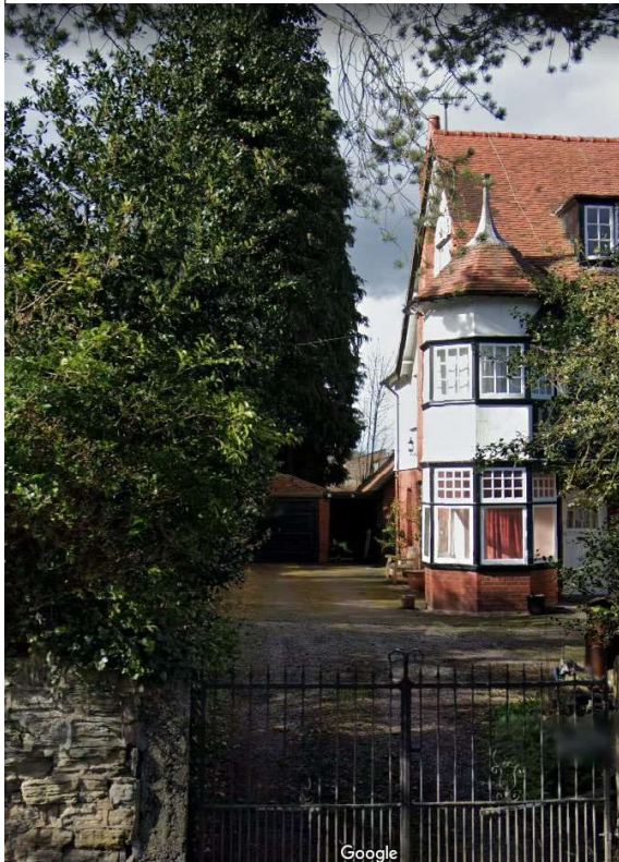
Photograph 2 - Turret Room on Ground Floor
